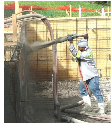
guncreting a pool
