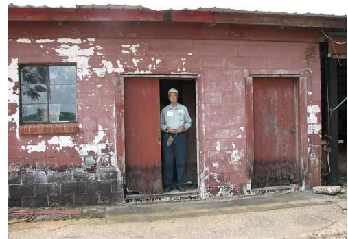
former Calhoun dairy
